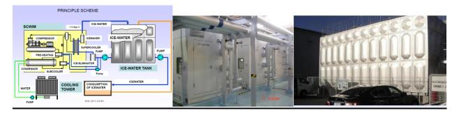
The principle scheme shows the 'SCWIM' supercooled water ice-maker, the ice-water tank with consumer circuit and the cooling tower.
