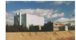
1993: Super GE (Superconduct- EL-Generator)
