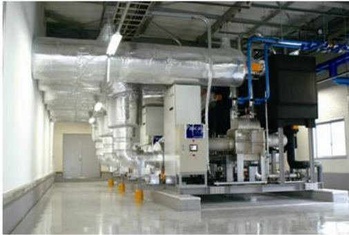
Figure 5 Installation of Pascal Air
