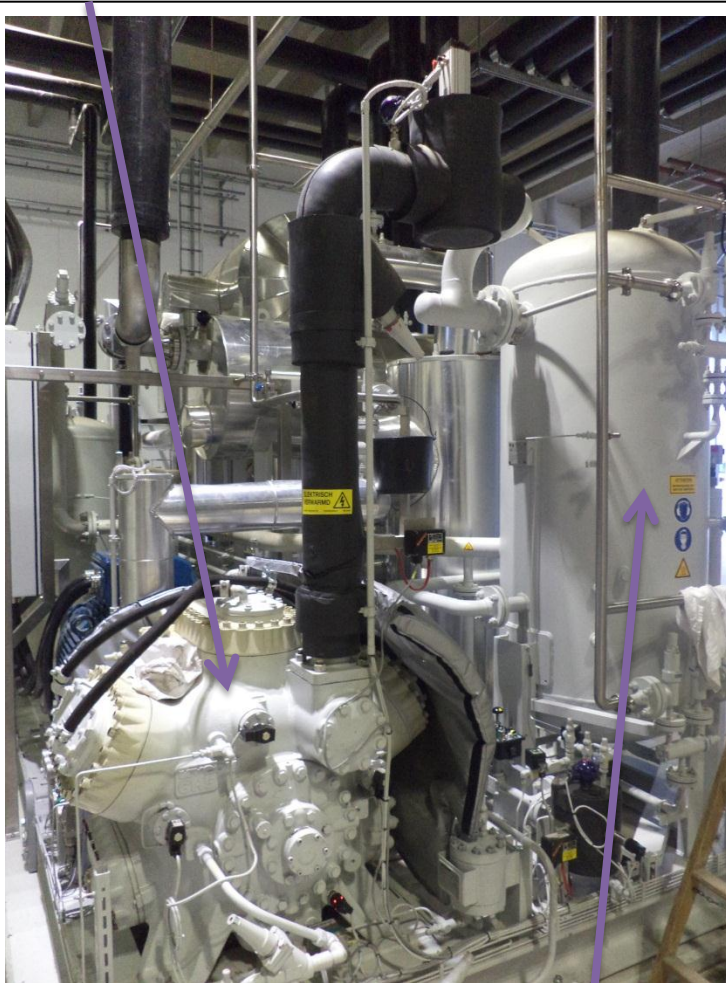
N6HS HIGH STAGE COMPRESSOR
