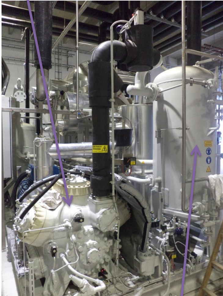
HEAT SOURCE FLASH TANK
